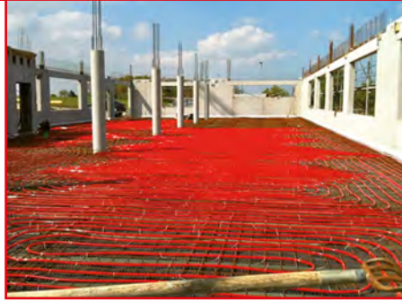
Installation of Underfloor Heating
